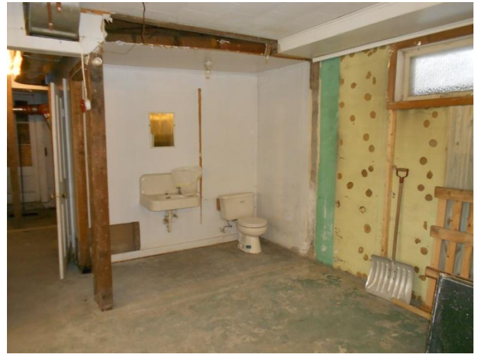
Removed walls await new ones
